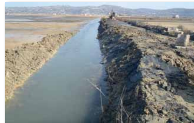
The dug out edge channels retain water in dry periods as well
